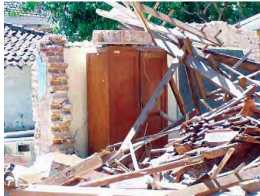
Figure 2.12 Collapsed school building in which furniture is still standing (Yogyakarta province, following Central Java Earthquake, 2006)
