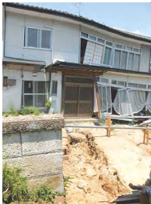
Figure 2.10 Houses damaged by failure of retaining walls
