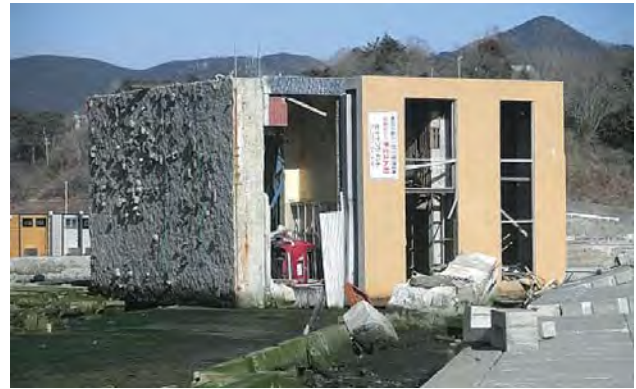
Figure 2.5 Reinforced concrete building damaged by buoyancy
