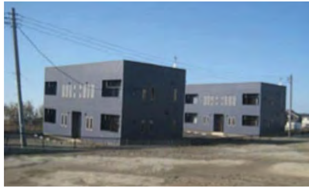
Figure 2.9 Subsidence of houses from liquefaction
