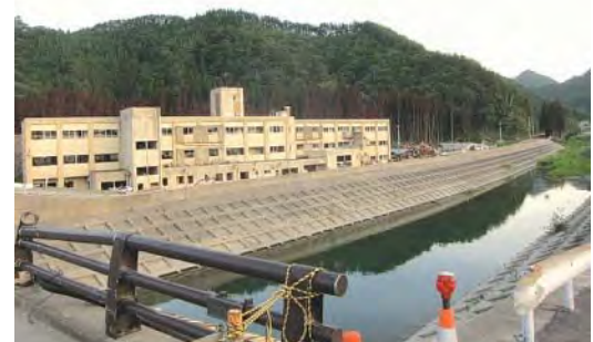
Figure 8.2 Kamaishi-higashi Junior High School (top) and Unosumai Elementary School (bottom) are located near the sea
