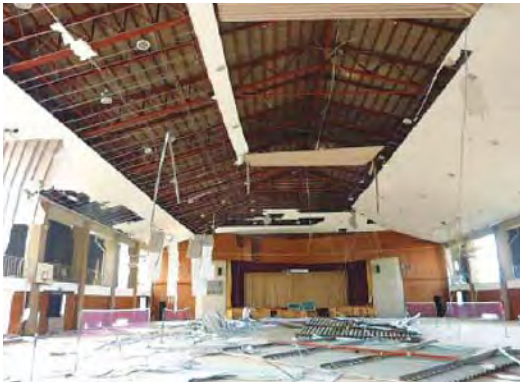
Figure 2.8 Fallen ceiling panels in school gymnasium
