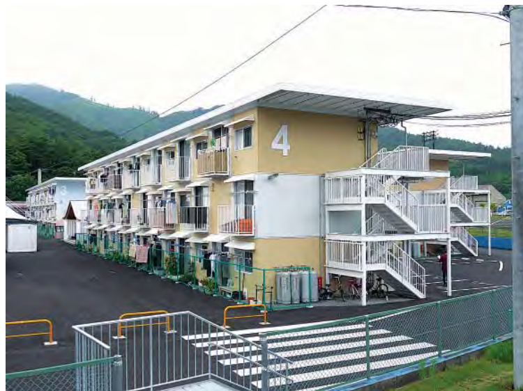
Figure 22.6 Multiple-story temporary housing made with stacked containers
