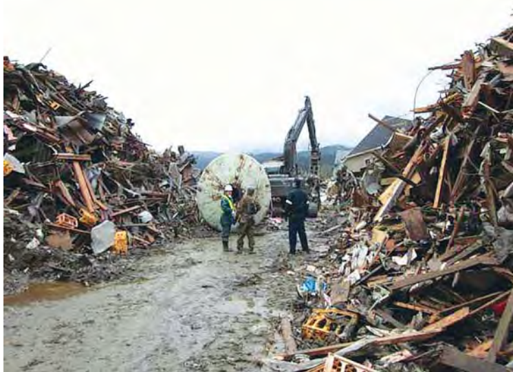
Figure 20.5 Clearing of roads
