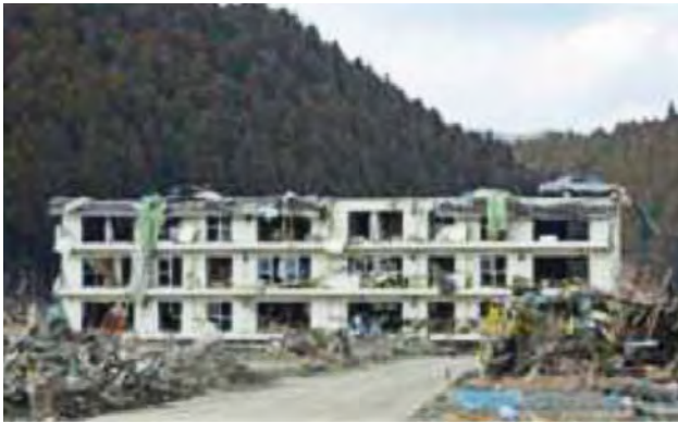
Figure 2.4 Reinforced concrete building withstood tsunami even though submerged (note car on roof)
