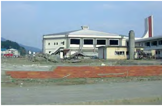
Figure 5.3 The Rikuzentakata City gymnasium
