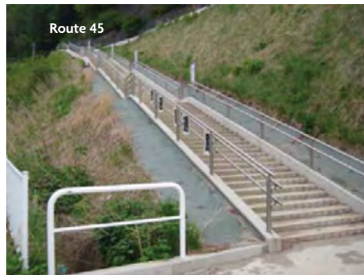
Figure 4.4 Evacuation stairway at the Omoto Elementary School
