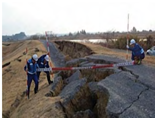
Figure 3.2 Damage to river dikes at Narusegawa
