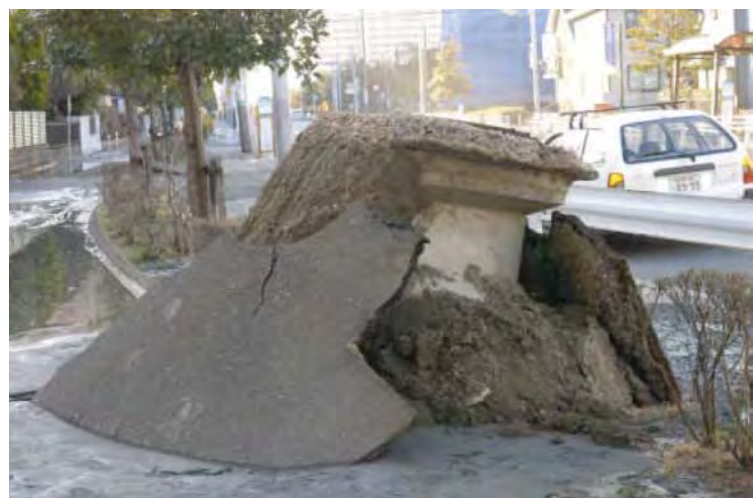
Figure 20.3 Manhole raised by liquefaction in Urayasu City
